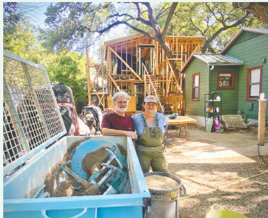
Susan Hays and contractor Carl Gradek building her hempcrete house in South Austin
