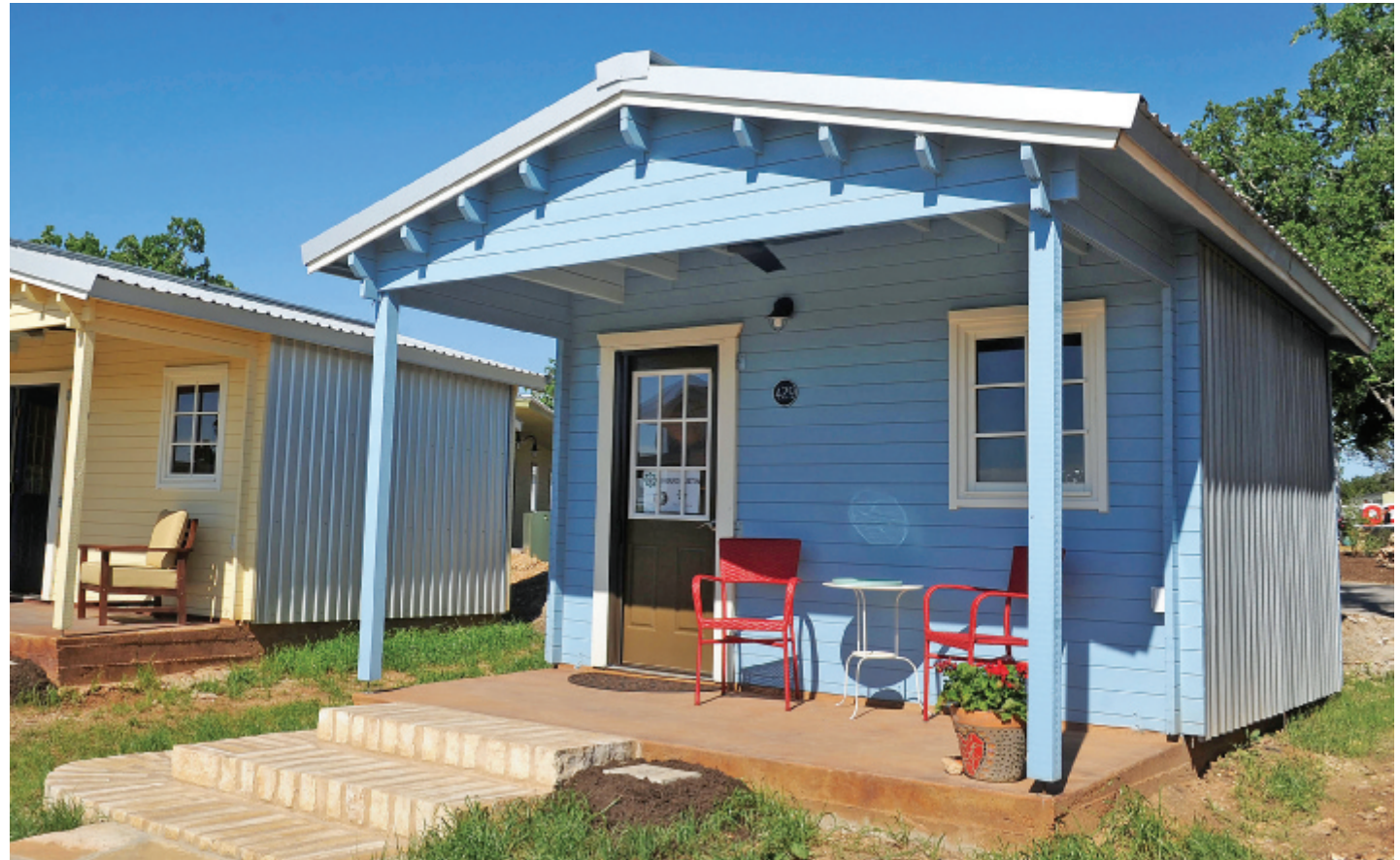
The city is in the midst of a push to make it easier to build tiny homes, duplexes, and triplexes
